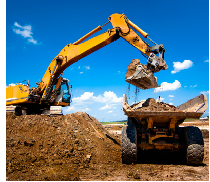
Figure 2: Corrosion can quickly develop on off-road equipment even in normal environmental conditions
